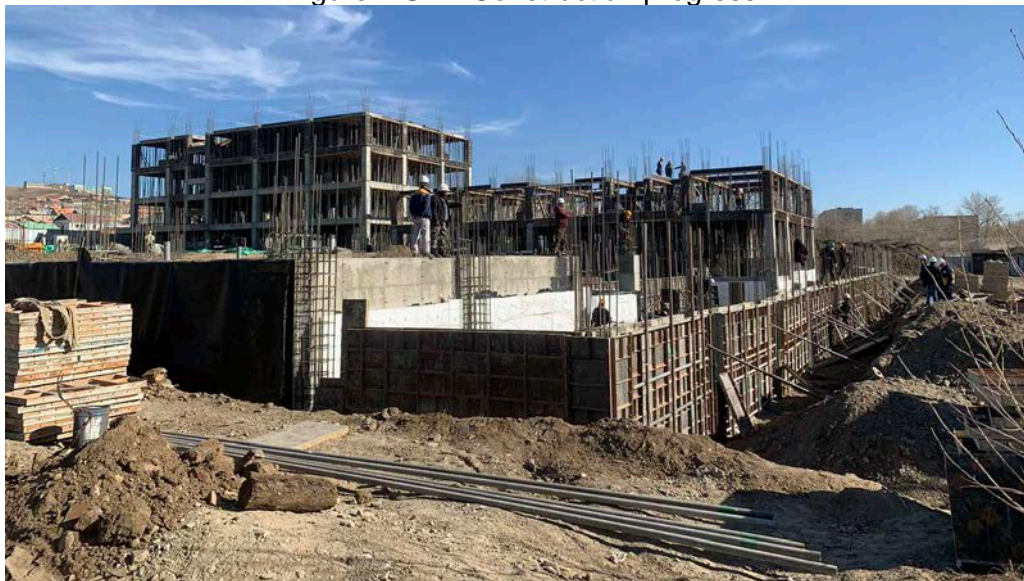
Figure 7 SKH Construction progress
